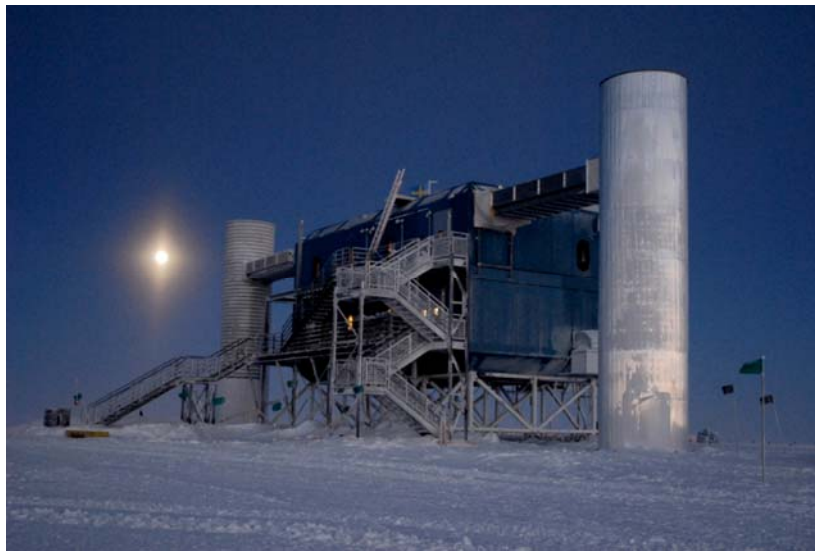
Figure 2. The new IceCube Control Station at the South Pole in March 2007. The outside temperature was -64°C
